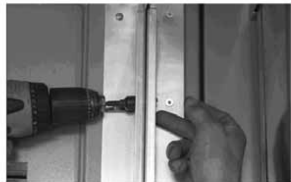
Figure 20. Connecting the corner posts
