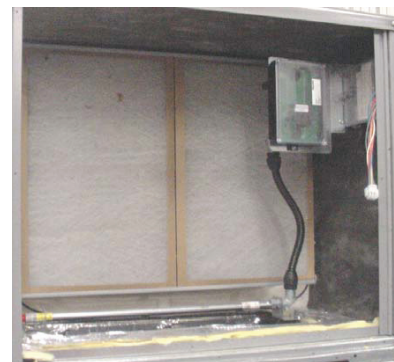
Fig. 38 - Return Air Sensor Operating Position
