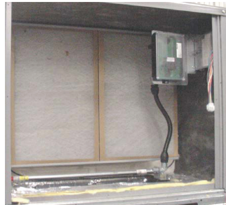
Fig. 40 - Return Air Sensor Operating Position
