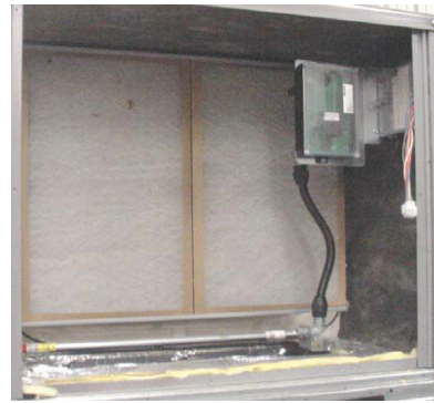
Fig. 34 - Return Air Sensor Operating Position
