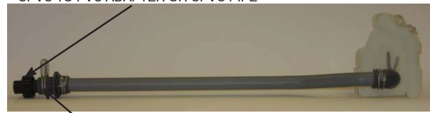
FRONT VIEW LEFT SIDE DRAIN PIPE ORIENTATION FOR CONDENSATE DISCHARGE NOTE: Remove Inducer Housing for easier access, if desired.
