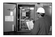
Generac RTS and HTS switches are open transition switches. Because load circuits can only be connected to one power supply at a time, open transition switches prevent electrical feedback between utility circuits and generator circuits.
