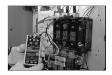
In any three-phase application, the phase rotation of the generator power lines must match the phase rotation of the utility power lines at the transfer switch.
