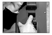
After the engine has completed its cooldown cycle and has shut off, open the main breaker and allow the generator to accept the entire load immediately. Verify gas pressure at the secondary regulator while the unit is under full load.
