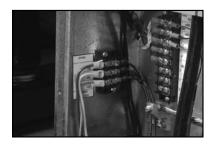
Connect the power leads for the battery charger to the 120-Volt, 15 or 20-Amp circuit as shown in the Installation Manual.
