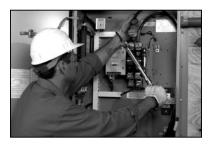
While supporting the lugs, use a torque wrench to tighten the lugs on the generator circuit breaker and the transfer switch. Torque specifications are in the Owner's Manual.
