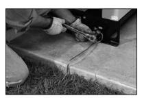
Connect an approved ground strap to the grounding lug on the base frame and to an earth ground or grounding rod consistent with local regulations.
