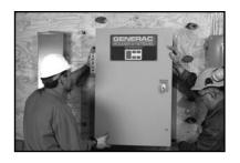
Always inspect the transfer switch for shipping damage. Never mount a switch that shows any evidence of damage.
