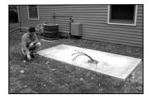
The length and width of the pad should exceed the length and width of the generator by at least 12 inches on all sides and the pad must be level within ½ inch all around.
