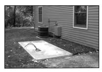
The mounting pad should be located as close as possible to the transfer switch and fuel supply. Make sure you leave adequate room around the generator for service access. Five feet is a good rule of thumb, but local codes vary.
