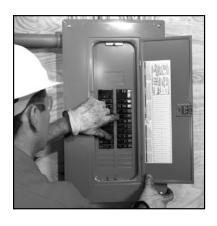
Make sure all breakers in the main distribution panel are open so that loads cannot be accidentally transferred to the generator until you are ready to do so.
