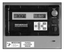
You'll need to check the control panel to make sure the H-100 controller is properly configured for the HTS transfer switch. Using the control panel is simple once you understand the process.
