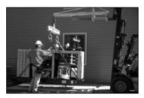
After removing the bolts holding the generator base frame to the wooden pallet, use the lifting eyes on the base frame to lift the generator onto the pad.
