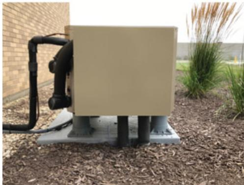
**Fig. 7 — Pipe risers installed**
