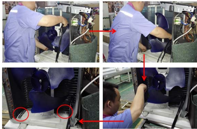
Fig. 4 – Install the Base Pan Heater
