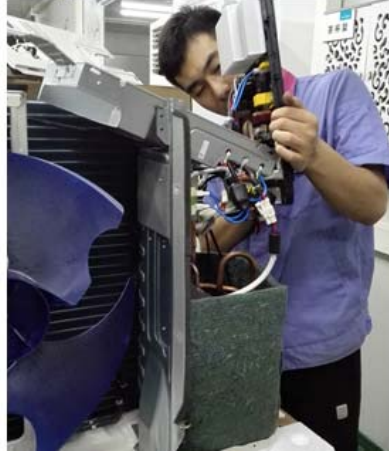
Fig. 3 – Replace the PCB Board
