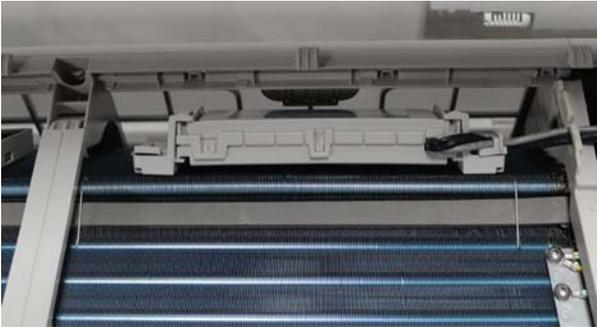
**Fig. 31 — Install the multi-function board**
