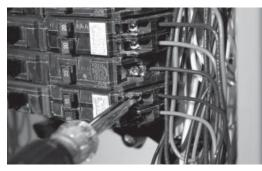
6. Next, connect the loads which are to be backed up. The breakers below the operator will be backed up by the generator during a power outage. Connect these loads to the appropriate sized breakers in the load center.
