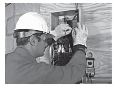
3. Energize the utility and check line-to-line and line-toneutral voltage at terminals N1 and N2 on the transfer contactor. If line-to-line voltage is not approximately 240 volts, de-energize utility power and check the terminations between the utility and N1 and N2.
