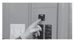
13. Shut OFF utility power and make sure the generator starts automatically after the line interrupt delay.
