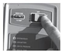
5. With the generator's main breaker OFF, put the mode switch in MANUAL to start the engine.
