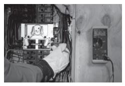
7. For all models except the 8 and 10 kW check to be sure that voltage from the generator is correct. If line-to-line voltage is not approximately 240 volts, refer to the generator Owner's Manual for the proper adjustment procedure. On all models, if line-to-neutral voltage is not 120 volts, check the neutral connection between the generator and load center.
