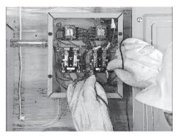
2. Using a multi-meter, make sure both the line and load sides of the contactors in the controller register 240 volts, and that the contactors are in the CLOSED position.
