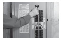
7. If the generator is not being installed at this time, loads can still be connected to the lower breakers. Simply make sure the utility feed breaker, the 2 pole breaker directly below the operator on the left side of the load center, is switched ON.
