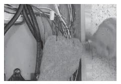
7. Choose a circuit to be backed up and remove the power lead from the breaker.
