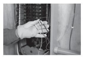
12. Remember that for every circuit moved from the main panel to the load center, the neutral will need to be relocated to the load center as well.
