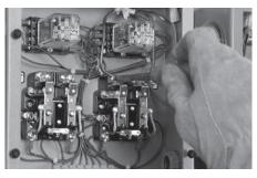
5. Connect the power leads that were removed from the appliance breaker to the load terminals in the controller.
