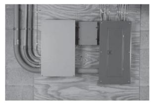
1. The PowerMaster load controller should be mounted as close to the main distribution panel as possible to avoid splicing. Refer to the instructions and wiring diagram in the PowerMaster Technical Manual before beginning the installation.
