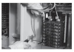
8. The grounding that is normally in the main panel must be accomplished in the Power Manager Load Shed transfer switch and must be disconnected in the existing distribution panel. Refer to the National Electrical Code (NEC) for complete information on grounding and bonding.
