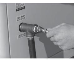
16. Unhook the gas meter and reinstall the port plug on the regulator.
