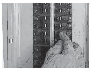
12. Shut OFF utility power again to automatically start the generator. When power has transferred to the generator, close each of the breakers in the distribution panel one at a time until the generator has accepted the entire load.
