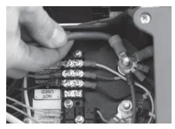
10. Connect the green equipment ground wire to the ground stud and torque to 100 inch lbs.
