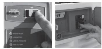
5. Put the generator's mode switch in MANUAL to start the engine.
