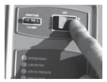
4. Put the generator's mode switch in MANUAL to start the engine. Allow the engine to warm up, then switch the generator's main breaker to the ON position. The generator is now supplying electricity to the transfer switch but is not carrying any load.
