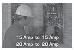
8. Using UL Listed wire nuts, reconnect the power lead to a matching breaker in the transfer switch.
