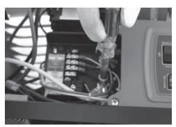
11. Connect the white neutral wire to the neutral post and torque to 100 inch lbs.
