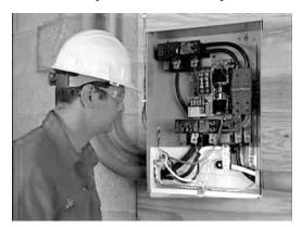
3. The grounding that is normally in the main panel must be accomplished in the service entrance rated switch and must be disconnected in the existing distribution panel. Refer to the National Electrical Code (NEC) for complete information on grounding and bonding.
