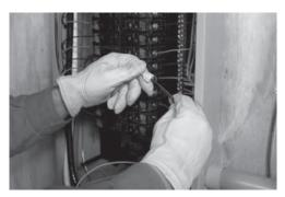
9. Make sure each circuit moved is protected by the same size breaker in the transfer switch. 15 Amp circuits must be connected to 15 Amp breakers and 20 Amp circuits to 20 Amp breakers.
