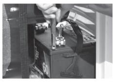
2. Follow all of the procedures and safety precautions in the generator Owner's Manual when installing the battery. Verify the switch is in the off position. When preparing for operational testing, DO NOT connect the battery until transfer switch connections are complete.
