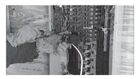
11. Install a 2-pole breaker in the distribution panel to protect the transfer switch. The required amp rating of the breaker depends on which transfer switch is used. If installing an 8-circuit, pre-wired load center switch, the breaker cannot exceed 40 Amps. For all other pre-wired load center switches the breaker cannot exceed 70 Amps. This breaker must be compatible with the existing electrical distribution panel.
