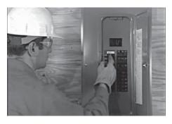
7. Make sure the 2-pole circuit breaker installed in the main distribution panel is in the OFF position.
