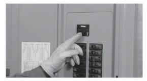
3. Switch the main utility breaker OFF and place all of the individual protected branch circuit breakers (located below the transfer operator) in the OFF position.
