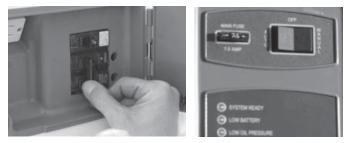
4. Switch the generator's main circuit breaker OFF and put the mode switch in the OFF position.
