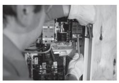
3. Connect the customer non-priority load leads to the E1 and E2 terminals on the load shed contactor.
