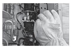
Locate the transfer handle, insert the metal end into the slot in the main contactor assembly and pull the handle DOWN to move the main contacts to the standby power, or generator position.
