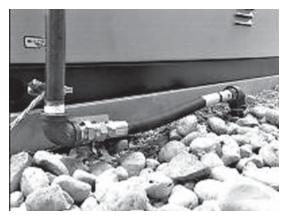
4. When connecting the gas line to the generator, use the provided section of UL Listed or AGA-approved flexible fuel line in accordance with local regulations. The purpose of the flexible fuel line is to ensure that vibration from the generator does not cause a gas leak at one of the connection points, so it's important that the line be installed with as few bends as possible.
