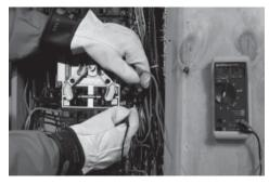
8. For 8 kW models check to be sure that the frequency from the generator is correct. If the frequency is not approximately 60Hz, refer to the generator Owner's Manual for the proper adjustment procedure.
