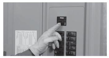
4. Make sure the central air conditioner will not start and simulate a power outage by shutting OFF utility power.
