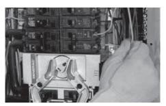
9. Connect the voltage sensing wires to the sense breaker. This is the 2 pole breaker directly above the operator on the right side of the load center. Connect N1 to one pole of the breaker, and N2 to the other.
