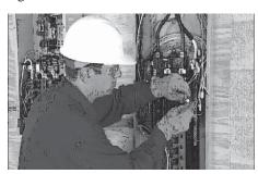
9. Make sure each circuit moved is protected by the same size breaker in the transfer switch. 15 Amp circuits must be connected to 15 Amp breakers and 20 Amp circuits to 20 Amp breakers.
