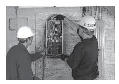
3. Protect against impact and mount the switch vertically to a rigid support structure. Make sure the switch is level and plumb.
