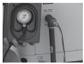
6. After checking for leaks, check the gas pressure at the T-fitting installed earlier to make sure there's enough pressure for proper generator operation.
