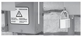
4. Replace the protective cover plate and retaining screw, and lock the connection box.
