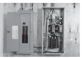
7. For all models except the 8 and 10kW check to be sure that output voltage from the generator is correct. If lineto-line voltage is not approximately 240 volts, refer to the generator Owner's Manual for the proper adjustment procedure. On all models, if line-to-neutral voltage is not 120 volts, check the neutral connection between the generator and transfer switch.
