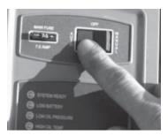
9. Now switch the generator's main breaker ON, and put the mode switch in AUTO.
