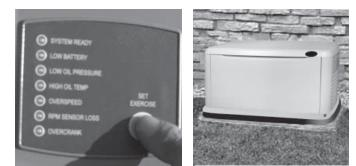
1. To set the exercise on 8 kW models, make sure with the mode switch is in AUTO. Press and hold down the EXERCISER switch for at least 10 seconds and release. The generator should start within a few seconds. The unit will run for about 12 minutes before shutting itself down automatically.
