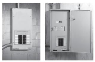
2. For applications with RTS Load Center switches and RTSS Load Shed transfer switches the charger has already been installed in the transfer switch. Discard the separately packed battery charger that came with the generator.
