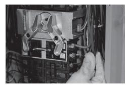
3. Connect the generator power leads to the generator feed breaker. This is the 2 pole breaker directly below the operator on the right side of the load center.
