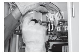
13. Connect the control wires from the generator to the terminal block in the transfer switch. The terminals are marked N1, N2, 23, 15B, and 0.
