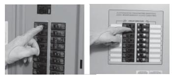
2. Next, make sure all of the individual circuit breakers in both the priority load center and in the non-priority sub-panel, are in the OFF position. If the sub-panel has a primary breaker, make sure it is in the OFF position as well.
