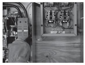
8. Connect one end of two control wires to the COMMON and NORMALLY OPEN pins on the generator side of the transfer switch.
