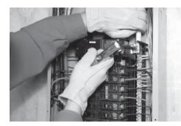
4. Be careful to support the lugs and torque the lugs in the transfer switch to the specifications shown in the transfer switch Owner's Manual.
