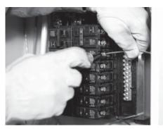
8. Reconnect the power lead to a matching breaker on the load center.
