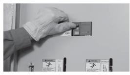
12. Switch the main breaker ON and make sure that power transfers back to the utility. The generator should shut down and go through a short cool-down cycle.
