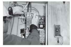
6. Check line-to-neutral voltage on N1 and N2. If voltage is not approximately 120 volts, de-energize utility power and check all of the neutral terminations between the utility and N1 and N2.
