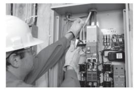
5. Neutral wires from the utility, generator and shedding panel are connected to the same neutral lug in the switch.
