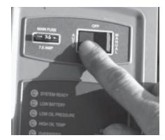
9. Using the mode switch, place the generator in AUTO. If utility power is still present, the generator will shut down.
