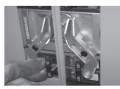
10. With utility power still OFF, switch the utility feed breaker (below the transfer operator on the left side of the load center) ON. This will also move the generator feed breaker to the OFF position.
