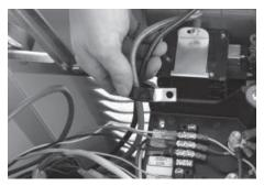
5. Run the power leads through the strain relief provided.
