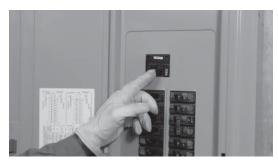
15. Shut OFF utility power again to automatically start the generator. When power on the lower half of the load center has transferred to the generator, turn ON each of the branch circuit breakers in the lower half of the load center, one at a time, until the generator has accepted the entire priority load.
