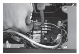
12. Connect the control wires to the correct terminals. The terminals are clearly marked N1, N2, 23 and 15B. If connecting a pre-wired switch a 0 (zero) wire will also be required.
