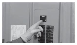
4. If not, switch OFF the main breaker, make sure all breakers and both contactors are in their correct positions and repeat the test.
