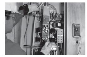
8. Check line-to-line voltage on terminals T1 and T2. If lineto-line voltage is not approximately 240 volts at any point in the system, switch the main breaker OFF and check terminations.
