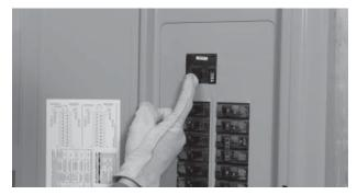
14. Switch the main breaker ON to restore utility power. The generator will continue to run to allow the engine to cool down before shutting itself off.
