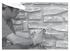
1. Drill a 1 <sup>3</sup>/<sub>4</sub> inch hole and feed the conduit through the hole.
