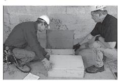
2. Always inspect the switch for shipping damage. Never mount a transfer switch that shows any evidence of damage.
