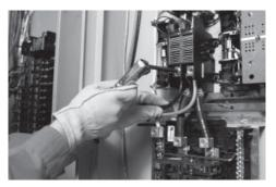
2. Connect the generator power leads to the E1 and E2 terminals on the transfer switch contactor.
