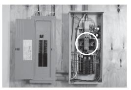
5. Make sure that both the main breaker and the primary sub-panel breaker are closed (ON), all branch circuit breakers are open (OFF) and that the contactors for both the transfer switch and non-essential load shed switch are in the UTILITY position.
