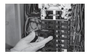
5. Connect the customer loads to the load center. The breakers above the operator are used for loads which will not be backed up during a power outage. Connect these loads to the appropriate sized breakers in the load center. When selecting circuits, note that the breakers immediately above and below the operator are dedicated for use by the generator and load center, and may not be used for customer loads.
