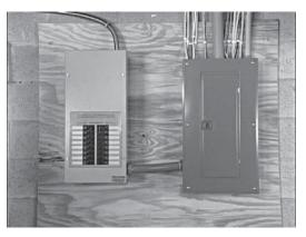
Before beginning any installation, make sure power is shut OFF to the main distribution panel and carefully read the Owner's Manual that came with the transfer switch. The distributed load center switch must be mounted close enough to the main distribution panel to accommodate the two-foot, pre-wired conduit. Make sure no water or corrosive substances can drip onto the transfer switch enclosure.
