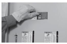
1. Before energizing utility power to the service, make sure the main breaker is in the open (OFF) position.
