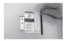
10. With utility power still OFF, use the transfer handle to move the main contacts to the UP (utility) position.
