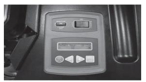
On all other models, the display will enter an Installation Assistant mode when battery power is first connected. The assistant will prompt to first enter the current date and time, followed by the exercise day and time. If the battery is ever disconnected and reconnected, or fuse removed and replaced, the Installation Assistant will be
