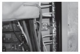
7. If the load center will serve as the service entrance for the house, install the ground to neutral bond. Refer to the National Electrical Code (NEC) for complete information on grounding and bonding.
