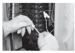
11. When moving two circuits with a shared neutral, they should be connected to adjacent positions (one above the other) on the load center. That will assure that the two hot wires are on separate phases and will maintain their relationship to neutral.
