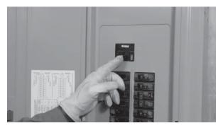
1. Switch the main breaker OFF. If there is a primary breaker in the sub-panel, make sure it is in the closed (ON) position.
