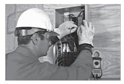
5. For all models except the 8 and 10kW check to be sure that voltage and frequency from the generator is correct. If line-to-line voltage is not approximately 240 volts, refer to the Owner's Manual for the proper adjustment procedures. On all models, if line-to-neutral voltage is not 120 volts, check the neutral connection between the generator and transfer switch.
