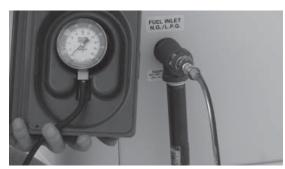
16. With the generator carrying the entire load, recheck gas pressure to verify that it's at the same level it was before the generator was started.
