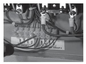
Connect the other ends of the control wires to the COMMON and NORMALLY OPEN positions of the selected control circuit in the controller. If moving a second load to the controller, follow the same procedure.
