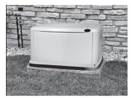
1. Locate the mounting area as close as possible to the transfer switch and fuel supply.
