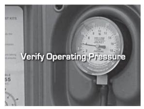
13. With the generator carrying the entire load, re-check gas pressure to verify that it's at the same level it was before the generator was started.
