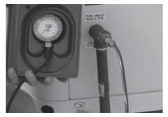
16. With the generator carrying the entire priority load, recheck gas pressure to verify that it's at the same level it was before the generator was started.
