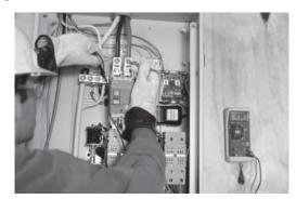
15. Close the Utility circuit breaker to restore utility power and make sure utility voltage at the transfer switch is correct. Refer to NFPA 70E for the safety equipment required when working inside a live transfer switch.
