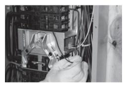
8. Connect the control wires from the generator to the load center operator. Connect the 23 wire to the XFER terminal, 15B to the BAT+ terminal, and 0 to the BAT-terminal.
