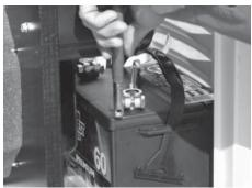
1. The generator was configured for natural gas operation at the factory. Switching over to LP Vapor is a simple procedure. On models with a single cylinder engine, begin by disconnecting and removing the battery if installed.
