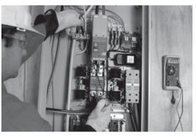
10. Make sure there is no voltage on terminals E1 and E2 at the transfer switch contactor. If voltage is present, switch the main breaker OFF and check the terminations.
