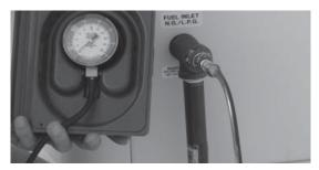
15. With the generator carrying either the entire load (or the priority loads if the non-priority loads were shed) re-check gas pressure to the generator to verify that it's at the same level it was before the generator was started.
