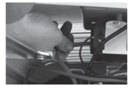
9. Now connect the red and black power leads to the circuit breaker. Since this is a single-phase application, it doesn't matter which wire is connected to which lug.
