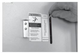
7. With utility power still OFF, use the transfer handle to move the main contacts to the UP (utility) position.
