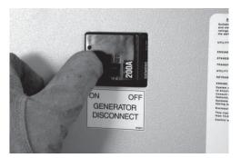
2. If using a service entrance rated transfer switch, put the generator disconnect switch in the ON position if applicable.
