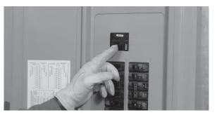
15. Shut OFF utility power again to automatically start the generator. When power has transferred to the generator, close each of the breakers in the distribution panel one at a time until the generator has accepted the entire load.
