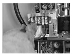
Connect the control wires from the generator to the terminal block in the transfer switch. The terminals are marked N1, N2, 23 and (194 or 15B). If the fourth terminal in the transfer switch is labeled 194, wire 15B from the generator will connect to terminal 194 in the transfer switch.
