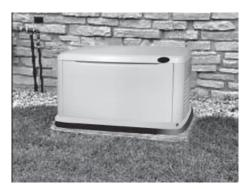
Set the generator onto the pad so that the gravel bed extends several inches beyond the generator on all sides. Make sure the generator is level within <sup>1</sup>/<sub>2</sub> inch.
