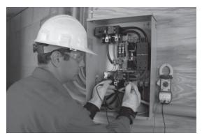
6. Check voltage and frequency from the generator. If line-to-line voltage is not 240 volts, refer to the Installation Guide for the proper adjustment procedures. If line-to-neutral voltage is not 120 volts, check the neutral connection between the generator and transfer switch.
