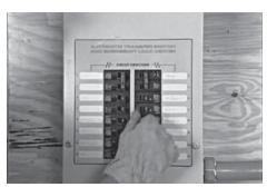
2. Make sure utility power is OFF and place all of the priority circuit breakers in the transfer switch in the OFF position.
