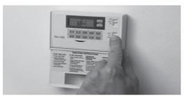
6. With the generator still carrying the load, start the central air conditioner.
