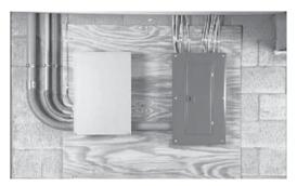
1. If installing the RTSE switch, the service was changed so make sure the terminations are good before re-energizing the utility.
