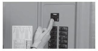
20. Close the main breaker to restore utility power and allow the engine to cool down and shut itself off.Operational tests are now complete. Refer to – Setting the Automatic Exercise Function to complete the installation.
