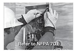
12. When all priority circuits have been moved to the transfer switch, close the main breaker to restore utility power and make sure utility voltage at the transfer switch is correct. Refer to NFPA 70-E for the safety equipment required when working inside a live transfer switch.
