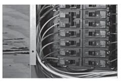
4. Each wire in the pre-wired transfer switch is color-coded to easily match circuits in the main panel to their new breakers in the transfer switch.
