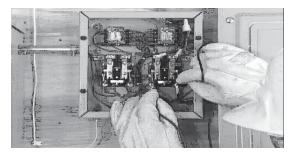
7. Check load side voltage again to be sure the selected appliances will not operate. Shut OFF the central air conditioner and re-check both line and load voltage to the selected appliances to be sure they are working again.
