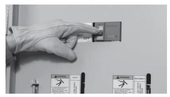
11. Shut OFF utility power at the transfer switch. The generator should start, and after a brief delay, the transfer contactor should move to the generator position.
