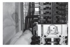
2. If the load center is being installed with a generator, locate and install the load center operator. Refer to the installation instructions packed with the operator for installation details.
