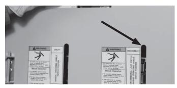
Next, insert the transfer handle into slot in the nonessential load shed switch assembly and move the contactor DOWN into the closed position.
