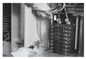
14. Complete the transfer switch wiring by connecting the equipment ground wire from the generator to the ground lug.
