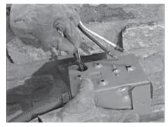
2. Remove the knockout in the back of the connection box, feed the wires through the back of the box and secure the conduit with the lock nut.
