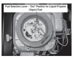
6. On all other models, simply remove the air cleaner cover and slide the fuel selector pin outward from the natural gas to the LP position.
