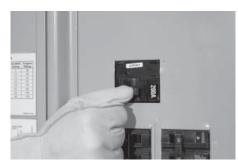
13. Shut OFF utility power at the main utility breaker and make sure the generator starts automatically.
