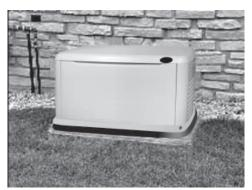
17. Shut OFF utility power again. The generator should start and the entire emergency load should transfer to the generator. Close the main breaker to restore utility power and allow the engine to cool down and shut itself OFF. If everything worked properly, the generator is now ready for automatic operation.
