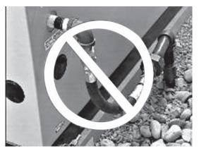
5. Never bend the flexible fuel line to avoid using an elbow. Bending the flexible line decreases its ability to absorb vibrations and defeats its purpose as well as constricts the actual fuel flow.
