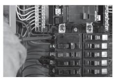
4. Connect the other end of the new power leads to the appliance breaker in the distribution panel.
