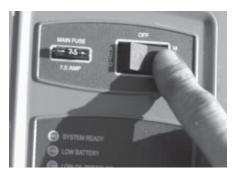
6. With the generator's main breaker OFF, place the mode switch in MANUAL to start the engine.
