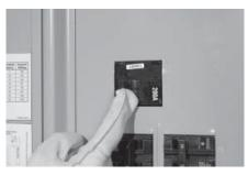
14. Switch the main utility breaker to ON and make sure that power on the lower half on the load center is automatically transferred back to the utility. This can be verified by noting the position of the utility feed and generator feed breakers.
