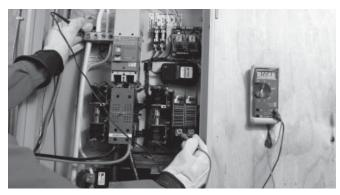
2. Make sure the use the transfer switch contactor is still in the UP (UTILITY) position, and use the transfer handle to move the non-essential load shed contactor UP to the open (SHED) position. To move the non-essential load shed contactor UP to the open (SHED) position.
