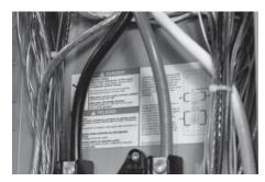
During installation, be careful to torque the lugs on all circuit breakers to the specifications listed in the load center Owner's Manual.
