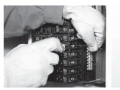
10. When three-conductor wiring is used, two 120 volt circuits will often share the same neutral wire. To avoid overloading the neutral, either move BOTH of the circuits that share the neutral or don't move either of them.
