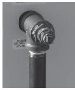
3. Where the gas line is to enter the generator, install a T-fitting to allow for gas pressure monitoring. On one opening of the fitting install a <sup>1</sup>/<sub>4</sub>" NPT nipple and threaded plug. In some cases a sediment trap may also be installed.
