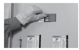
7. With all branch circuit breakers still OFF, close the main breaker by switching it to the ON position.
