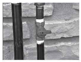
7. When finished checking the gas pressure, close the manual shutoff valve.
