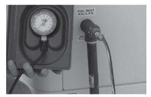
13. With the generator carrying the entire priority load, recheck gas pressure to verify that it is at the same level it was before the generator was started.
