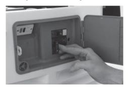
Manually switch the generator circuit breaker (just below the transfer operator) to the ON position. This will also move the utility feed circuit breaker to the OFF position. NEVER MOVE THE LOAD CENTER FEED BREAKERS MANUALLY WHEN LOADS ARE CONNECTED.
