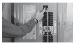
2. Switch the generator's main circuit breaker OFF and put the mode switch in the OFF position.
