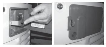
5. For 10-20 kW models, locate the metal hasp that is packaged in the owner's manual bag. Insert the hasp in the slot located on the left side of the external circuit breaker box. Be sure that the clip of the hasp is facing toward the front of the generator. If desired, lock the external box.
