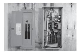
6. The transfer switch being used is an open transition switch. Open transition switches prevent electrical feedback between the generator and the utility by only allowing load circuits to be connected to one power supply at a time.
