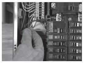
2. After making sure that all power supplies are shut off, remove the power leads from the 240 volt, 2-pole breaker that controls the selected appliance.
