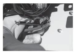
4. Feed the wires through the back of the generator and secure the conduit with the lock nut.
