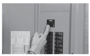
3. With all branch circuit breakers still OFF, switch the main breaker ON. The load shed contactor should automatically move DOWN to the closed position, verifying that the load shedding switch is working properly.
