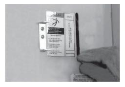
6. Locate the transfer handle, insert the metal end into the slot in the main contactor assembly. Pull the handle DOWN to move the main contacts to the standby power (generator) position.
