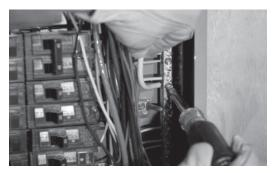
4. Connect the neutral wire from the utility and generator to the neutral bar on the right side of the load center panel and the generator equipment ground wire to the ground bar on the left side of the load center panel.
