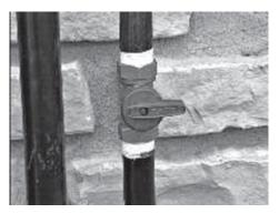
2. Most applications will require an external manual shutoff valve on the fuel line.
