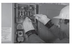
5. When the generator is carrying the entire load, check the voltage on the load side of the contactors to be sure the appliances connected to the controller are working properly.
