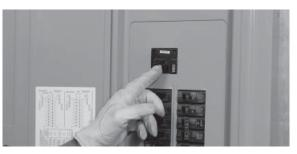
10. Shut OFF utility power and make sure the generator starts automatically.
