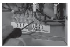
6. Now run 24 volt control wires from the air conditioning circuit to the terminal strip in the controller.
