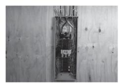
4. Protect against impact and mount the load center vertically to a rigid support structure. Make sure the load center is level and plumb.
