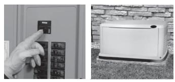
10. Shut OFF utility power and make sure the generator starts automatically.
