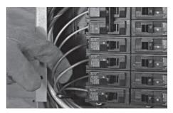
6. When moving two circuits with a shared neutral, they should be connected to adjacent positions (one above the other) in the transfer switch. That will assure that the two hot wires are on separate phases and will maintain their relationship to neutral.
