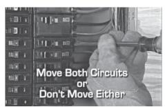
5. When three-conductor wiring is used, two 120 volt circuits will often share the same neutral wire. To avoid overloading the neutral, either move BOTH of the circuits that share the neutral or don't move either of them.
