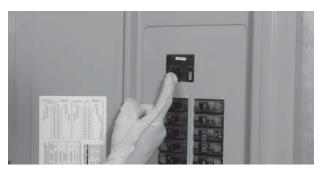
14. Switch the utility breaker to ON and make sure that power is automatically transferred back to the utility.
