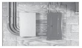
Before beginning any installation, make sure power is shut OFF to the main distribution panel and carefully read the Owner's Manual that came with the transfer switch. To simplify the installation process, the transfer switch should be mounted as close to the main distribution panel as possible. Make sure no water or corrosive substances can drip onto the transfer switch enclosure.
