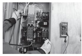
11. Next, check the voltage to the load shedding switch.
