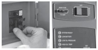
1. Switch the generator's main circuit breaker OFF and put the mode switch in the OFF position.
