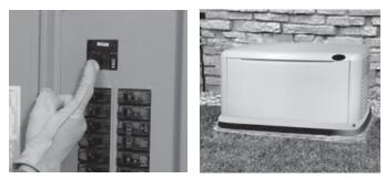
11. Switch the utility breaker to ON and make sure that power is automatically transferred back to the utility.
