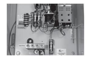
1. The battery charger is to be installed in the generator when using an RTSN or RTSE transfer switch. Refer to the Battery Charger Installation Guide for details.
