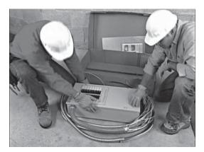
Always inspect the switch for shipping damage. Never mount a transfer switch that shows any evidence of damage.
