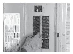
3. Make sure utility power is OFF and place all of the individual circuit breakers in the main distribution panel in the OFF position.
