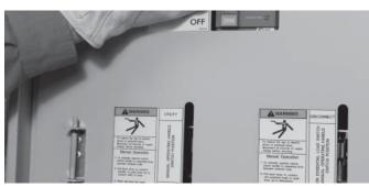
3. Locate the yellow transfer handle, insert the metal end into the slot for the transfer switch contactor assembly and move it UP into the UTILITY position.
