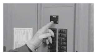
2 Switch the main utility breaker OFF. Refer to NFPA 70-E for the safety equipment required when working inside a live transfer switch.
