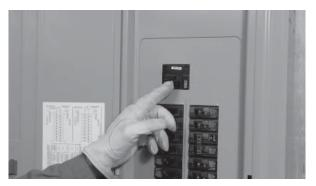
13. Now check the terminations in the sub-panel. If there is a primary breaker in the sub-panel, make sure it is in the OFF position. Then check line-to-line and line-to-neutral voltage at the primary breaker.
