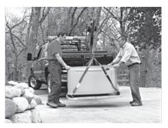
4. Make sure the lifting equipment to be used has sufficient capacity to safely handle the weight of the generator. Use nylon lifting straps and connect them to the lifting eyes on each corner of the base frame to avoid damaging the enclosure.
