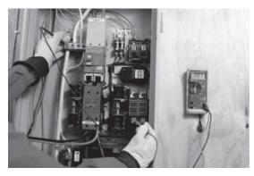
12. Check both line-to-line and line-to-neutral voltage on terminals E1 and E2. Terminations to T1 and T2 were made at the factory, but still make sure that voltage is correct at these terminals.
