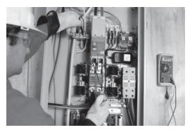
9. Next, make sure line-to-neutral voltage at T1 and T2 is approximately 120 volts. If line-to-neutral voltage is not approximately 120 volts at any point in the system, check neutral terminations.
