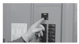
18. Shut OFF utility power again. The generator should start and the entire load should transfer to the generator. If the load is too large, the non-essential load shed switch will automatically shed the non-priority loads.
