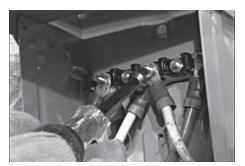
3. Mount the connection box so that it completely covers the hole in the wall. Caulk around the sides and top of the box to ensure a good seal.
