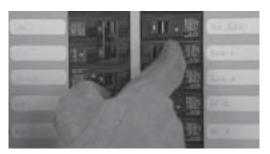
After the engine has completed its cool down cycle and shut down, shut OFF utility power again.
