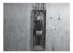
6. The load center being used contains, or will contain, an open transition operator. Open transition prevents electrical feedback between the generator and the utility by only allowing load circuits to be connected to one power supply at a time.
