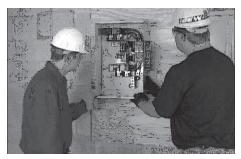
3. Protect against impact and mount the switch vertically to a rigid support structure. Make sure the switch is level and plumb.
