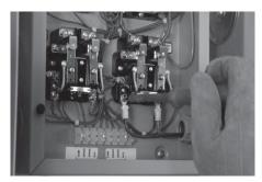
3. Using the ring lugs provided and the wire specified in the PowerMaster Technical Manual, connect one end of new power leads to one of the contactors in the load controller.
