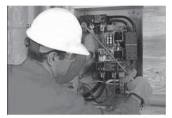
5. Being careful to support the lugs, torque the lugs in the transfer switch to the specifications shown on the transfer switch. Decal located on the inside of the switch door.
