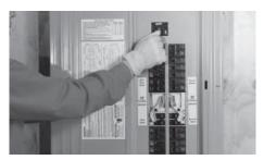
10. Switch ON the main utility breaker if not already on and switch on the utility supply breaker for the priority circuits. Make sure utility voltage at the load center is correct. Refer to NFPA 70E for the safety equipment required when working inside a live load center.
