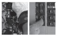
8. Use the transfer handle to move the main contacts in the transfer switch to the UP (utility position). Switch the 2-pole breaker ON in the distribution panel.
