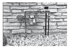
Both natural gas and LP Vapor are highly volatile substances, so strict adherence to all safety procedures, codes, standards and regulations is essential. Gas line connections should be made by a certified plumber familiar with local codes. Always use AGAapproved gas pipe and a quality pipe sealant or joint compound.
