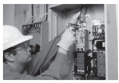
1. Connect the utility power leads from the meter to the Utility circuit breaker in the transfer switch.
