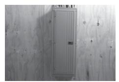
1. Before beginning any installation, make sure power is shut OFF and carefully read the Owner's Manual that came with the load center.
