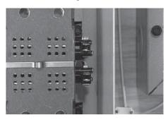
7. The auxiliary switches that came with the controller must be installed in the transfer switch. These switches ensure that the controller will only disconnect the selected appliances when utility power is off and the generator is running. Refer to the Technical Manual for specific instructions for installing the auxiliary switches.
