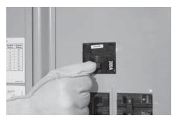
5. With the main breaker OFF, energize the utility and check the voltage at terminals N1 and N2 on the transfer contactor. If utility voltage is not approximately 240 volts, de-energize utility power and check all of the terminations between the utility and N1 and N2.
