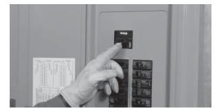
5. Make sure utility power is OFF and place all of the individual circuit breakers in the main distribution panel in the OFF position.
