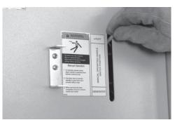
4. Locate the transfer handle and insert the metal end into the slot in the main contactor assembly. Pull the handle DOWN to move the main contacts to the standby power (generator) position. NEVER OPERATE THE TRANSFER SWITCH MANUALLY WHEN LOADS ARE CONNECTED.
