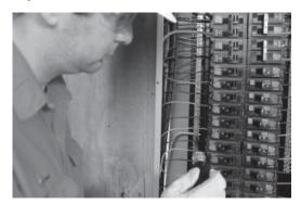
7. Select a priority circuit to be backed up and remove the power lead from the breaker.
