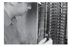
6. In this step, move priority load circuits, which will always be backed up by the generator, from the existing electrical distribution panel to the 16 circuit load center in the Power Manager Load Shed switch.
