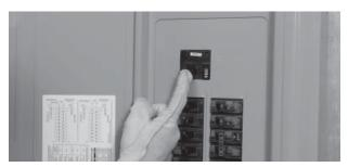
11. If everything worked properly, switch the main breaker to ON and make sure that power is automatically transferred back to the utility.
