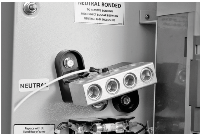
Figure 3.5 — RTSE Neutral Connection
