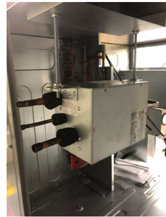
Fig. 49 - FS Unit Mounted to Threaded Rods
