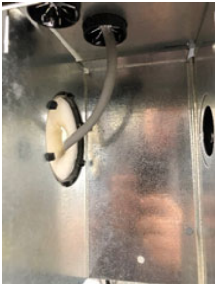
Fig. 58 - Route Wire Through Bottom of Control Box
